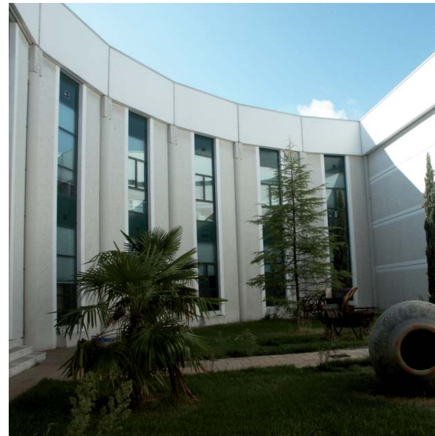
Blanco Mármol with framing finish por panels and Gris Liso for enclosure walls
