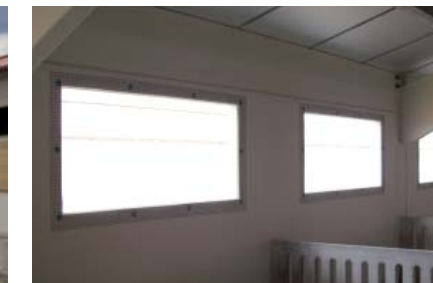
Interior fly screens on windows and attachment of dividers to walls
