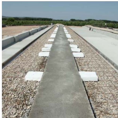
3 | Graded aggregate in aisles.
