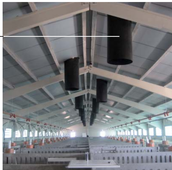
Ventilation system by means of ventilation shafts
