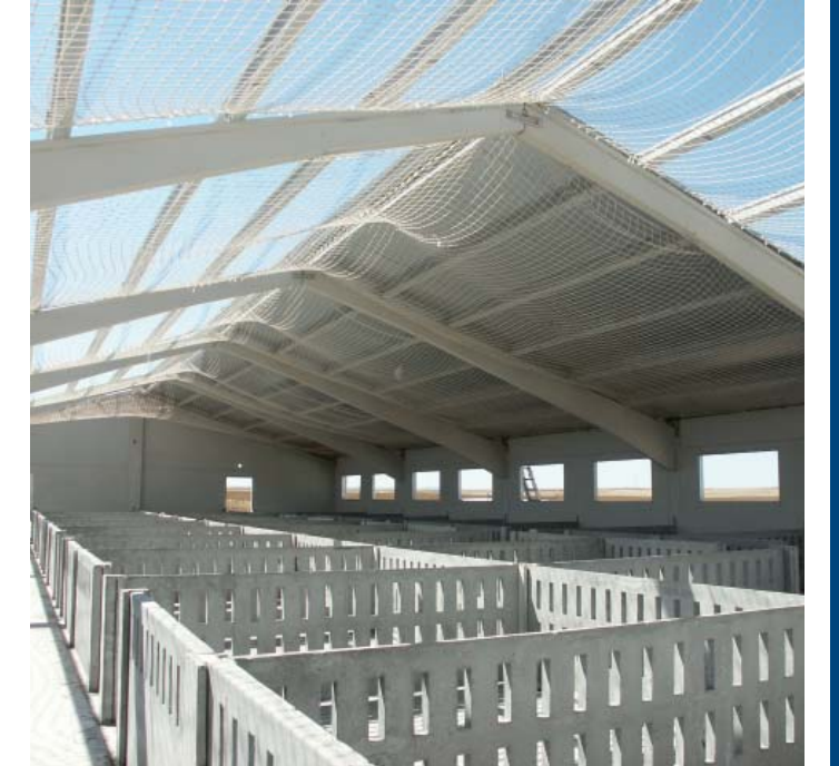
Partial mounting of roof viewed from inside
